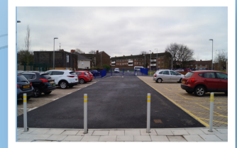
Visitors car park
